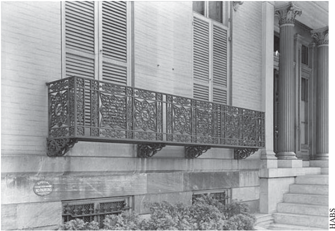
Cast iron balconies, Mt. Vernon, ca. 1851
