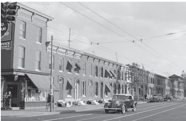
Awnings in historic Baltimore, c. 1940.
