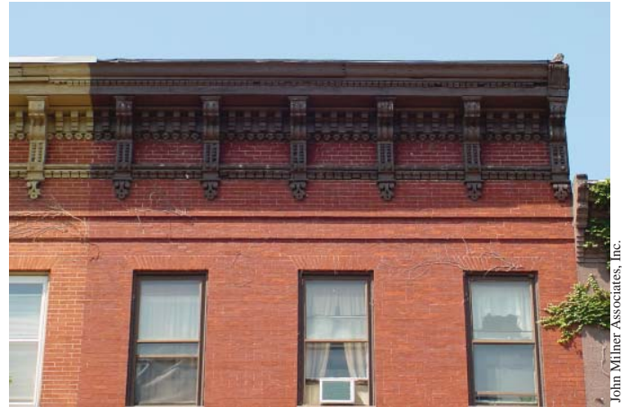
Typical wood cornice at Italianate rowhouse
